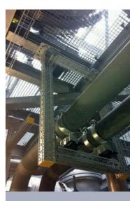
Archive photo: Modular bolted siFramo system for rapid assembly of secondary steel constructions
