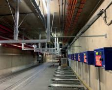
The geothermal ring pipeline is 1,500 m long, with nominal pipe sizes from DN 100 to DN 500 mm, and Sikla delivered more than 25,000 kg of material to secure it. The materials included 1,100 m of TP F 80 beam sections, 400 m of TP F 100 beam sections, 14,000 FLS F self-locking screws and 350 Simotec pipe shoes.
